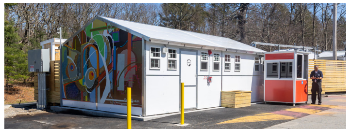
Level concrete pad for Community 400
