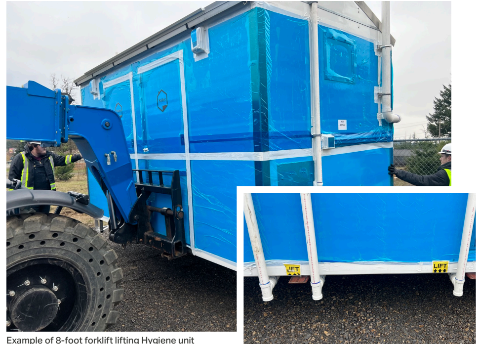
Example of 8-foot forklift lifting Hygiene unit
